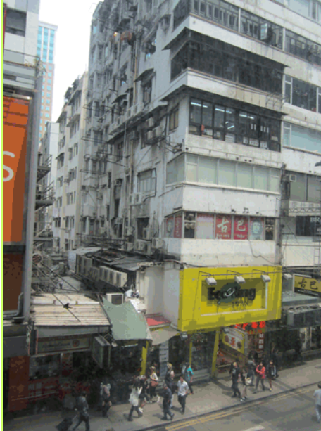
Photo A - Typical Kowloon structure!
